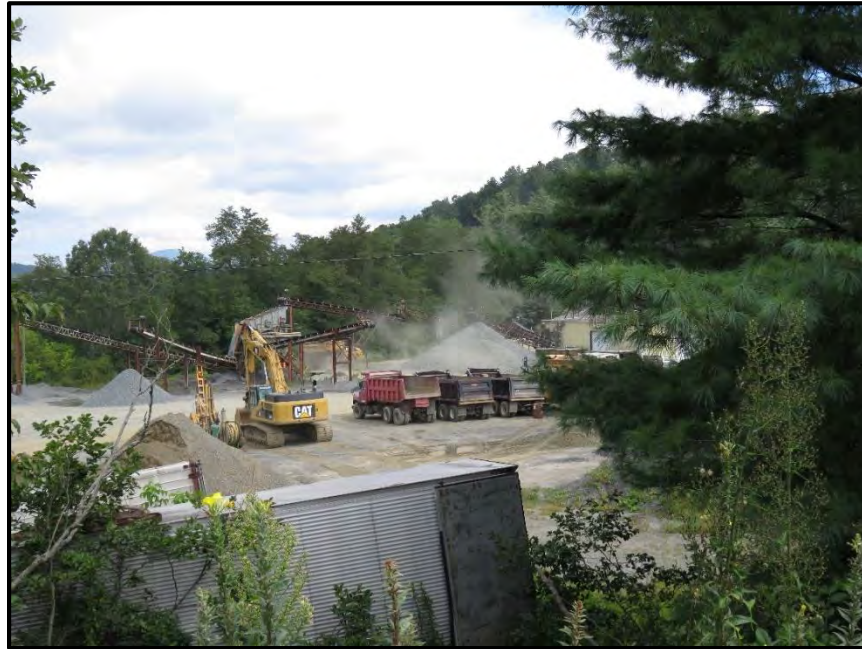
Figure 20: Overview of the western section of the property with dump trucks alongside the equipment building, looking northeast.
