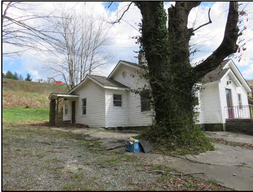
Figure 7: Corner view of the former residence, looking southeast.
