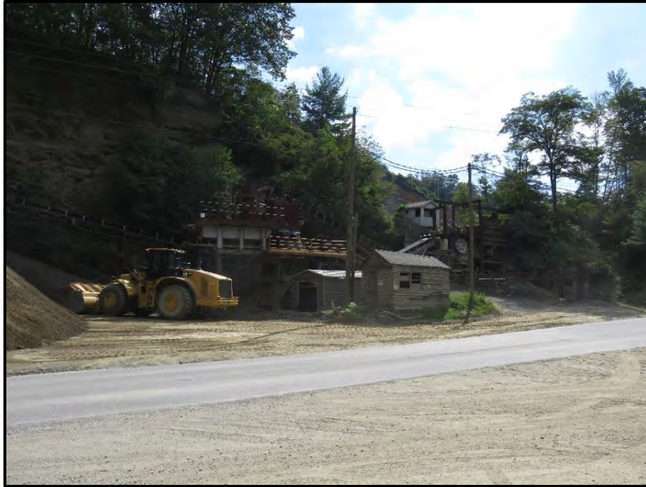
Figure 12: Overview of WT950 quarry machinery as visible from the ROW, looking southeast.
