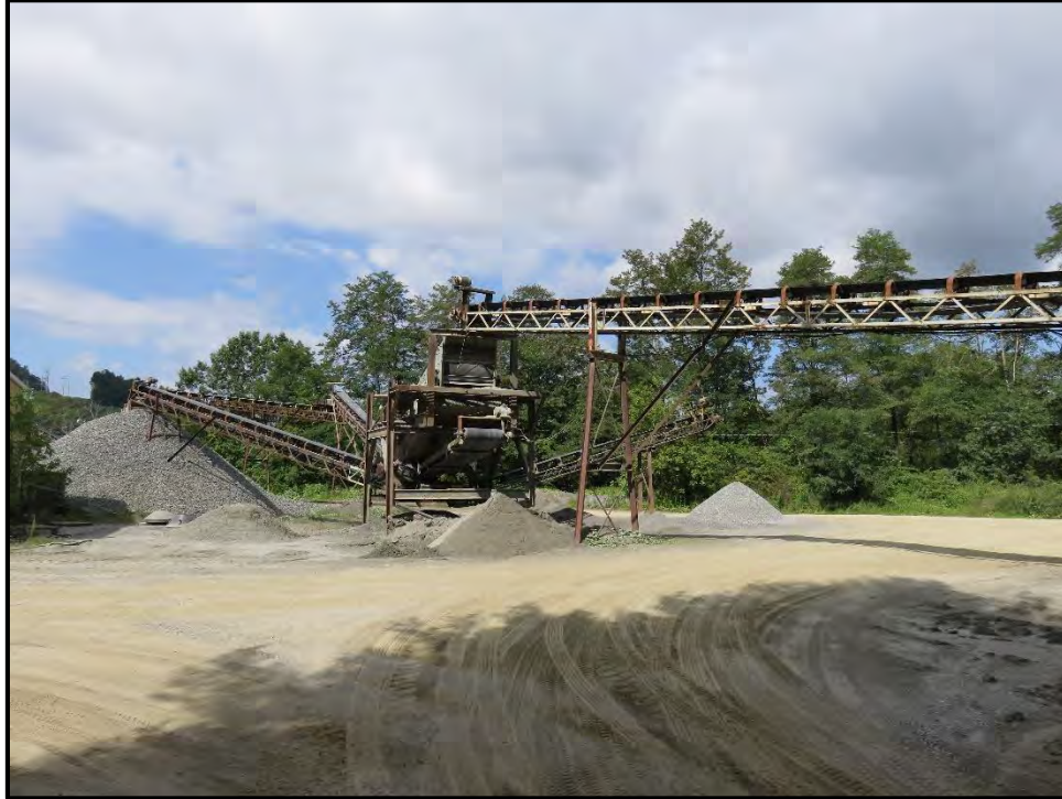
Figure 18: Northwestern view of second crusher, looking northwest.
