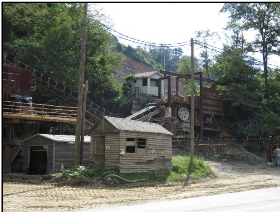
Figure 11: Detail view of sheds, looking southeast.
