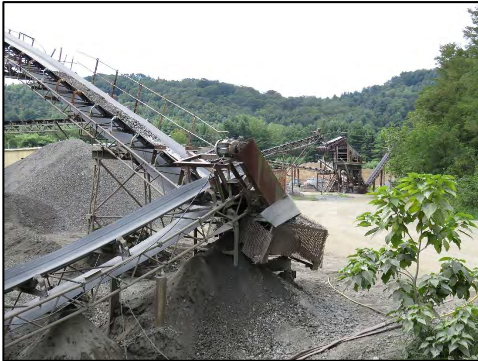
Figure 15: View of the belts connecting both crushers, looking west.
