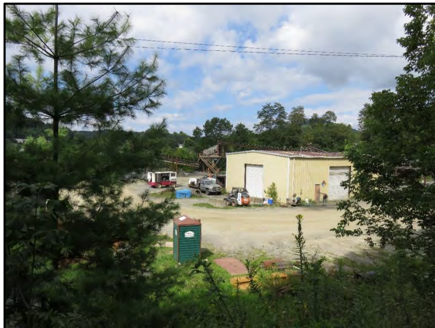
Figure 21: Western view of the equipment building, looking northeast.
