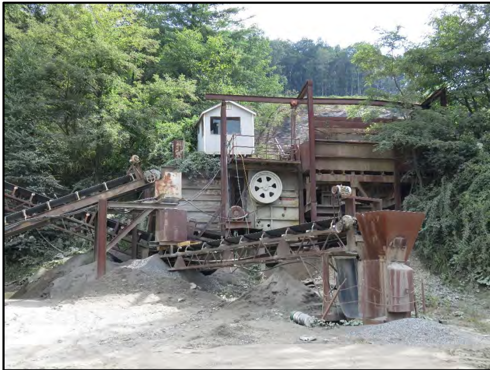
Figure 10: View of quarry machinery with Cedarapids jaw crusher, hopper, conveyor belts, and operator observation shed, looking east.
