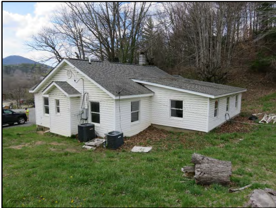
Figure 8: Rear view of the former residence, looking northwest.
