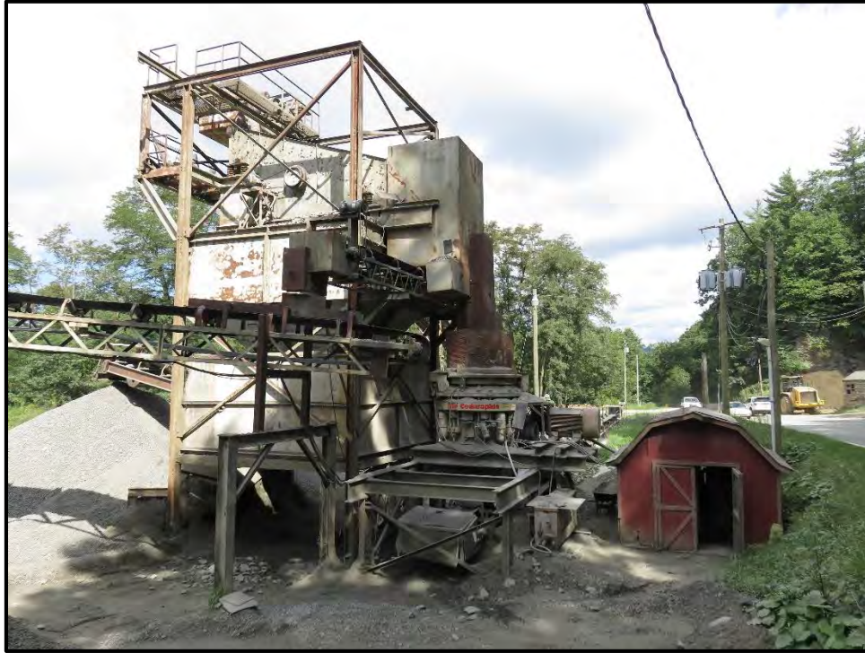
Figure 16: View of the prefabricated shed and crusher, looking north.
