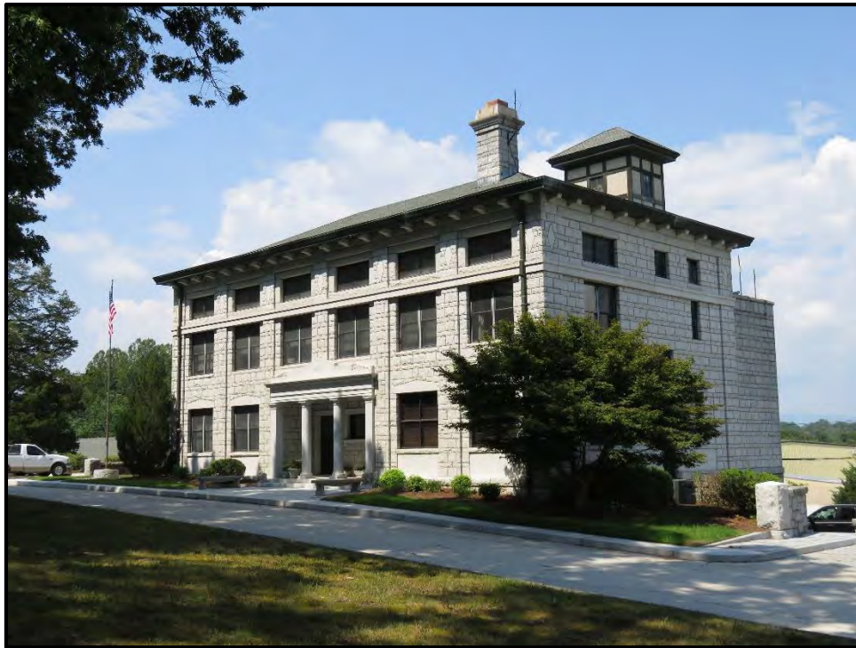
Figure 23: North Carolina Granite Corporation quarry office building constructed in 1928, looking west.
